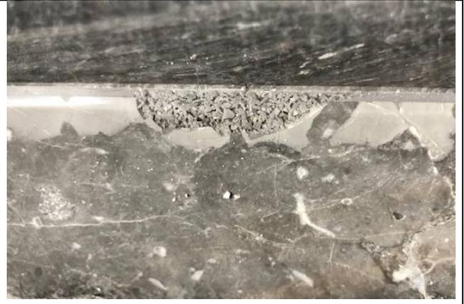
EXAMPLE OF HAND MADE REPAIR WITH RESIN AND MARBLE GRAINS ALONG TABLE EDGES
