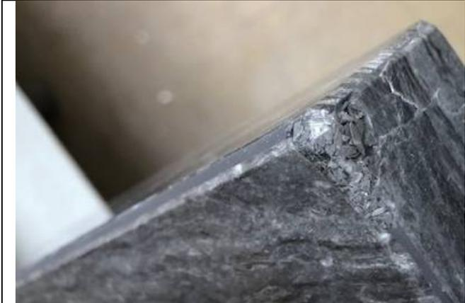
EXAMPLE OF HAND MADE REPAIR WITH RESIN AND MARBLE GRAINS AT TABLE CORNER
